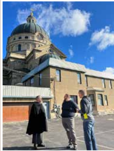
Fr. Jim with members of the parish discussing the upcoming renovations of the parking lot of the Basilica.
